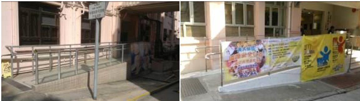
Resurface of the ramp way to reduce risk of slip/fall
